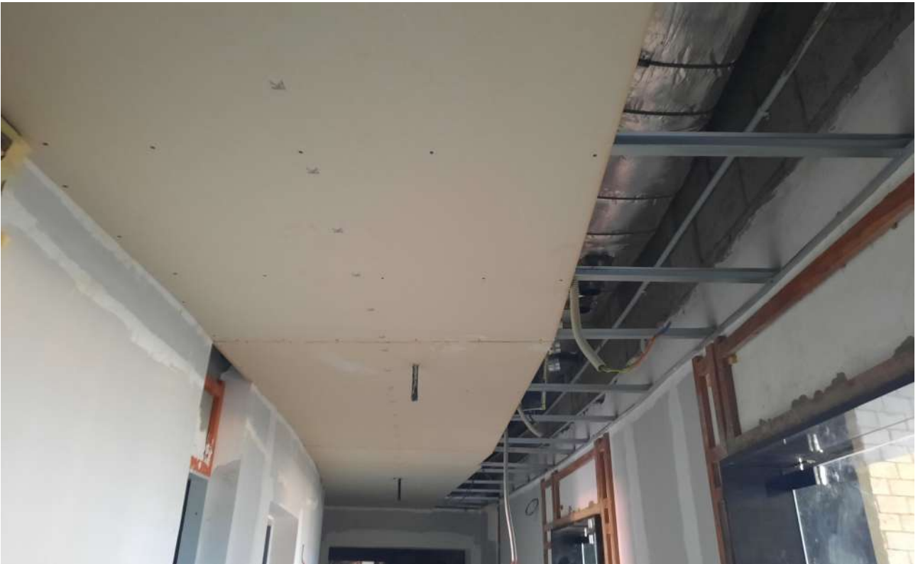
False Ceilling at Corridor (Ground Floor)
