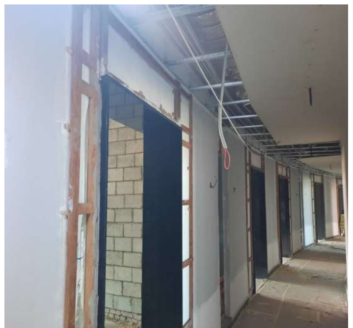
False Ceilling at Corridor (Ground Floor)
